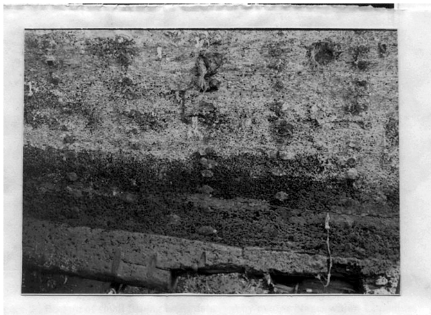
Fig. 1 Keel and side planks of a teakwood boat, showing severe destruction by marine wood-borers. Note the intensity of infestation. (Locality: Panaji, Goa)
