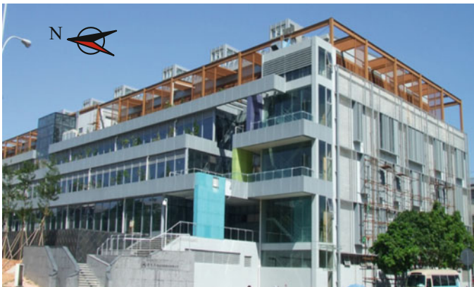
Fig. 8.10 The tested office building in Shenzhen
