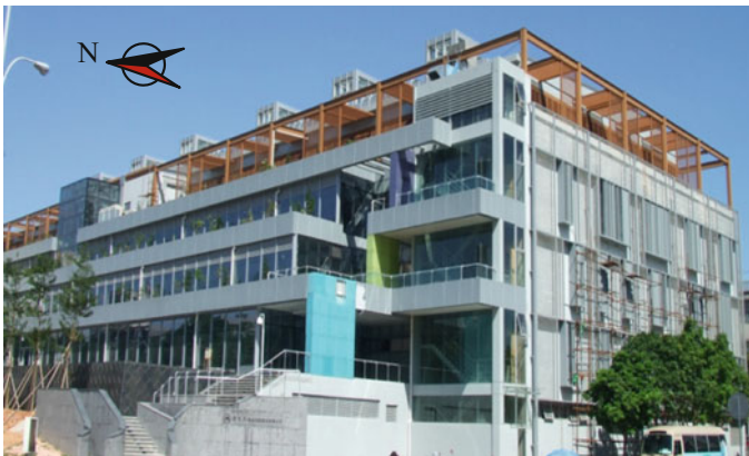
Fig. 8.10 The tested office building in Shenzhen
