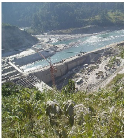
Dam Site Over Teesta
