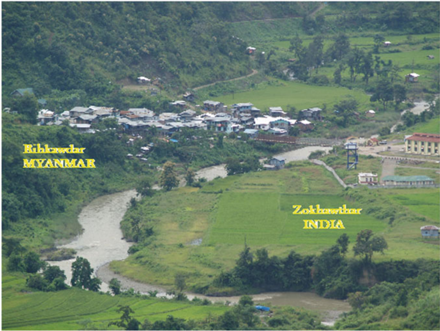
Tio River Bridge at Indo Myanmar Border, Mizoram
