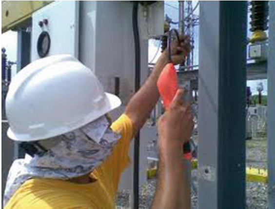
Fig. 6.15 SF6 gas leakage detector
