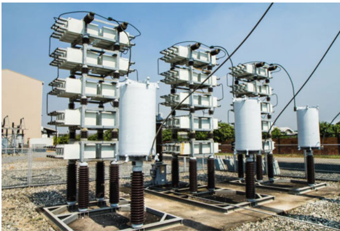
Fig. 4.3 Capacitor bank
