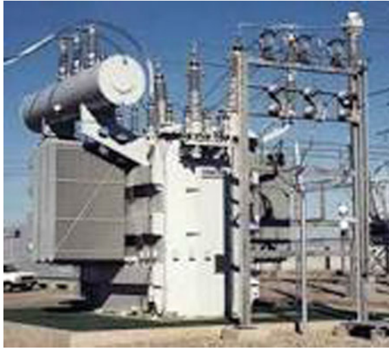
Fig. 5.1 Power transformer
