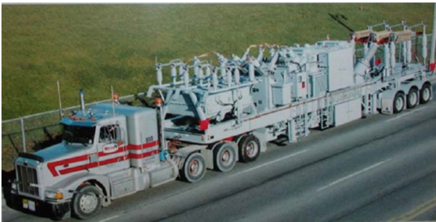
Fig. 7.3 Mobile substation in transit
