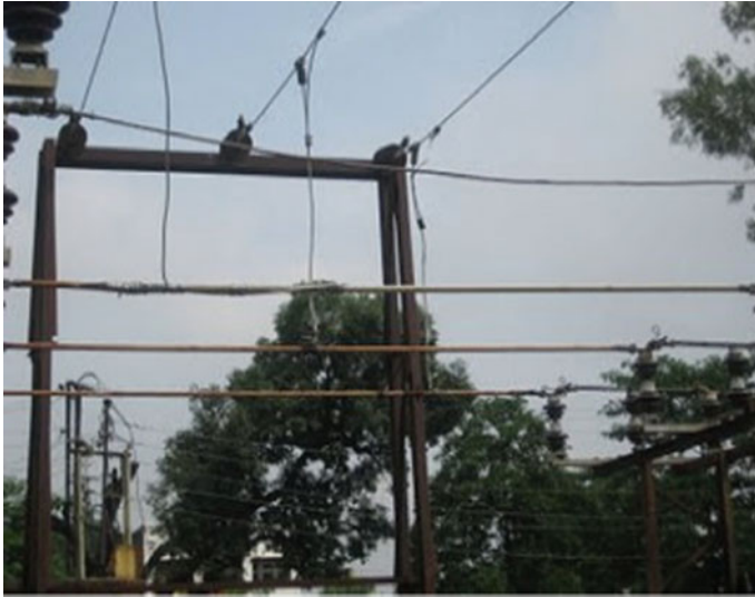
Fig. 4.4 Bus bar arrangement
