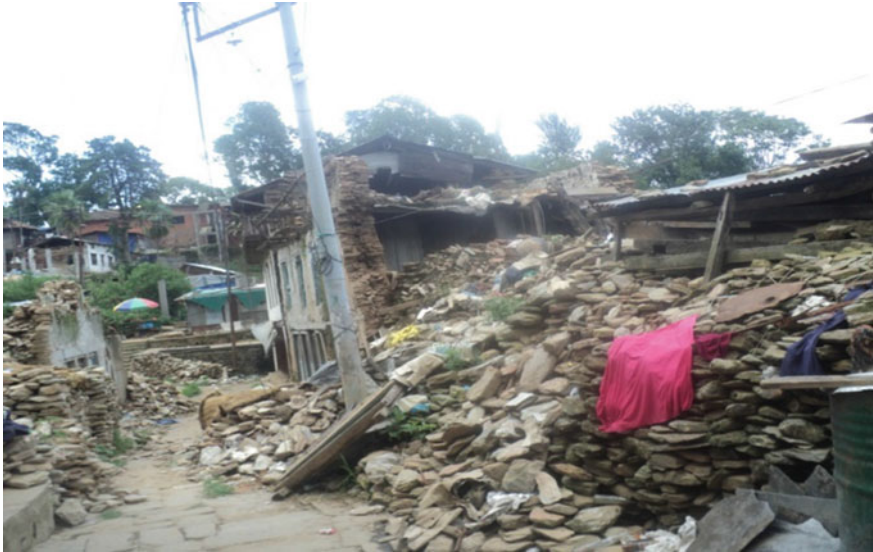
Fig. 20.5 Earthquake devastation in Dolakha
