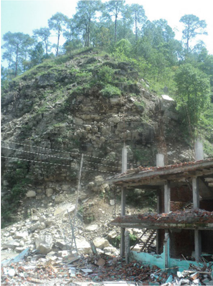
Fig. 20.4 Landslides in Singati due to earthquake
