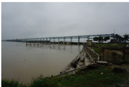
Koshi river barrage (Photo by Bo Kong)
