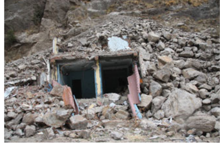
Destroyed building by landslide induced by 4-25 Earthquake (Photo by Xi Nan)
