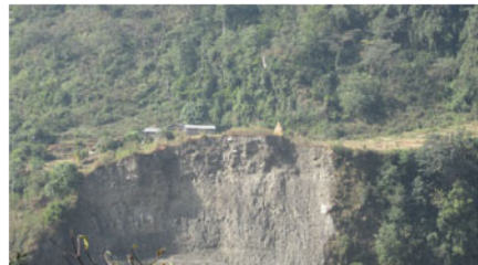
The house few meter away from the landslides (Palunge, Machhapuchhre VDC, photo by Prabin Poudel)
