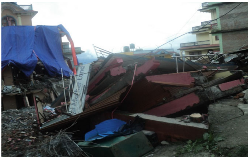
Fig. 20.7 Collapsed building of Charikot bazaar
