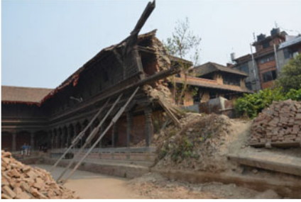
Old building destroyed by 4-25 Earthquake in bhaktapur durbar square (Photo by Jifei Zhang)
