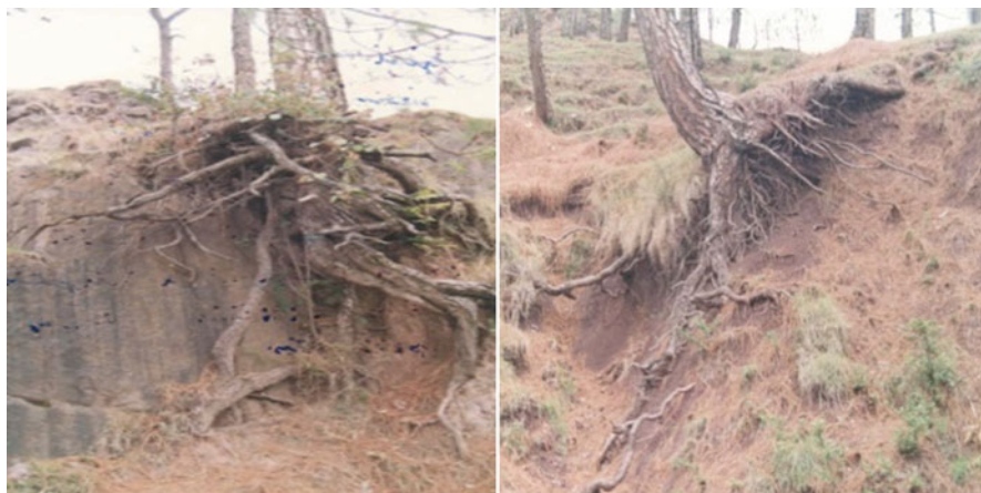
Fig. 15.3 Exposure of tree roots as a result of soil erosion
