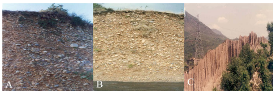
Fig. 15.4 Man-made soil erosion (a, b) due to road cut in Shivalik. (c) Severely eroded Shivalik hills on Bilaspur–Shimla road
