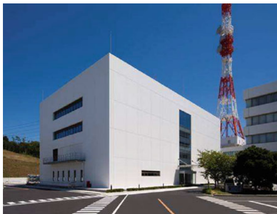
Fig. 10.15 Seismically isolated office building ( Photograph Chubu Electric Power Company )
