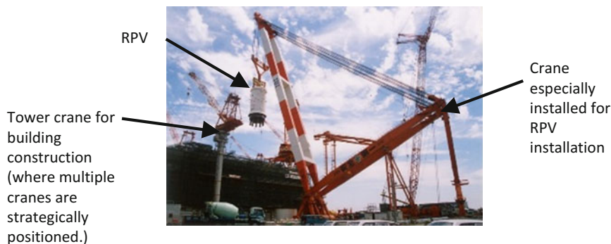
Fig. 10.7 RPV hoisting (Photograph Chubu Electric Power Co., Inc.)
