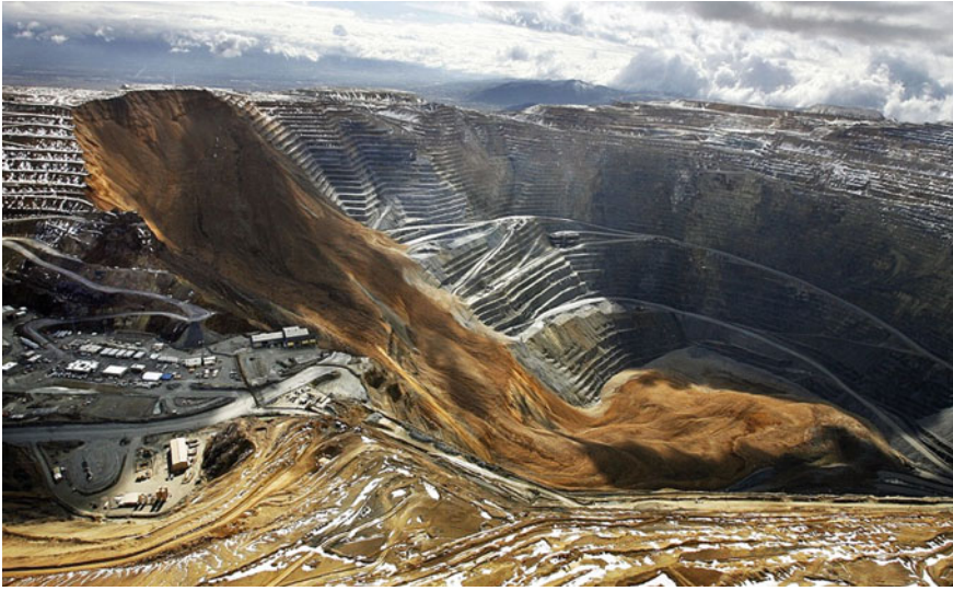
Fig. 6 A devastating landslide at the Bingham Canyon Mine outside of Salt Lake City, Utah (Source Daily Mail UK, 1 June 2013)
