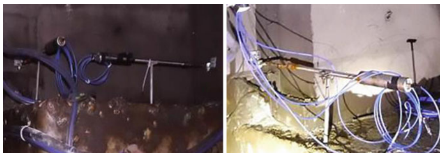
Fig. 8 The installation of the FBG sensor
