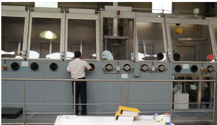
Fig. 5 Equipment photograph of dry waste sorting box, precompactor, and shearing box
