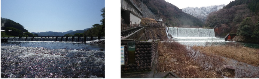
Photo. 2. Yoshii Weir (left panel) and Hinobori Weir (right panel) installed in the mainstream of Hii River.
