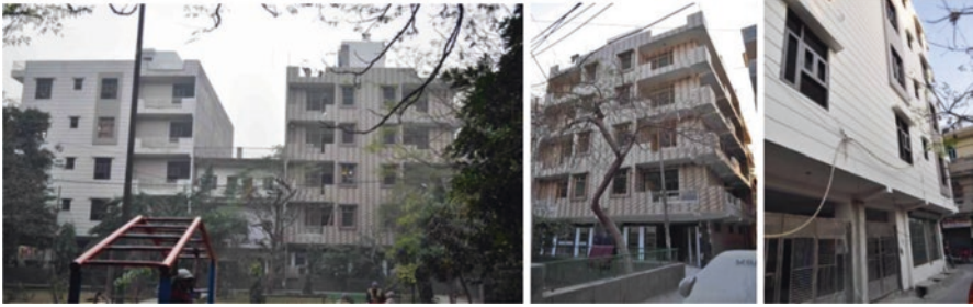
Figs. 4.2, 4.3, and 4.4 Photographs showing the newly built builder floors in the colony
