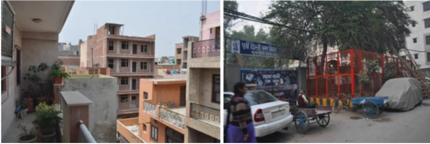
Figs. 4.12 and 4.13 (On the left ) A builder floor under construction and (on the right ) social infrastructure in study area
