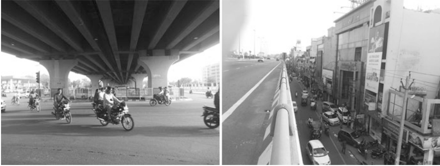
Fig. 5.8 Panipat flyover: segregation of regional and local traffic
