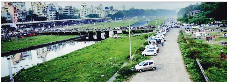
Fig. 15.5 Channelization of Mutha River in Pune (Source: Clicked for personal use)
