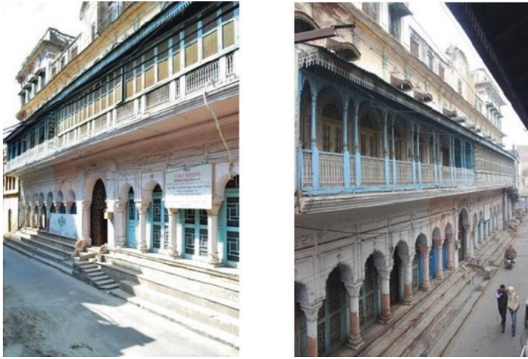
Fig. 14.6 Verandahs on southern side for reducing solar radiations
