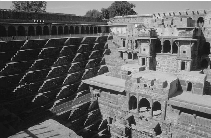
Fig. 8.1 The Chand Baori at Abhaneri is a subterranean hydraulic structure to access subsoil water
