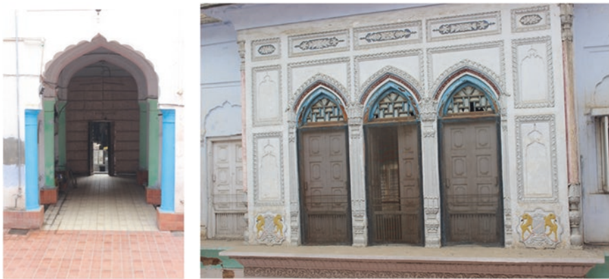
Fig. 14.7 Covered passage to connect two courtyards and balcony above opening
