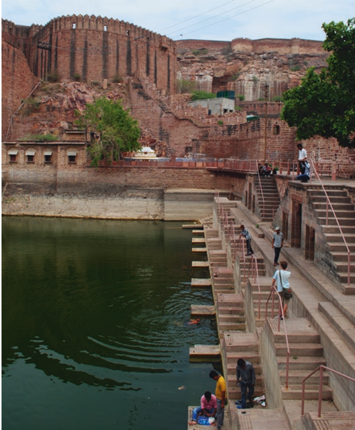
Fig. 8.2 The Ranisar at Jodhpur collects water from the surrounding hills by damming a narrow part of the valley. The bund, with its steps to access water, becomes a public space for the city. It provides water to the fort seen in the background through a system of wells, pulleys, and channels
