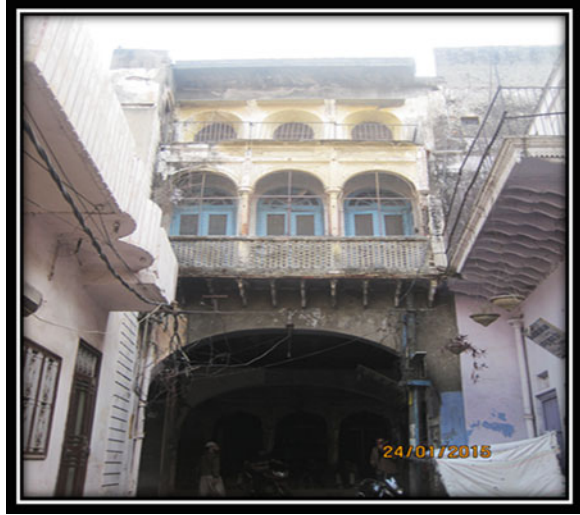
Fig. 18.7 A general view of chhatta Barumal
