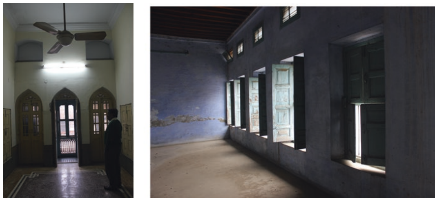
Fig. 14.8 Recessed openings provide sufficient glare-free daylight and ventilators near ceiling create stack effect
