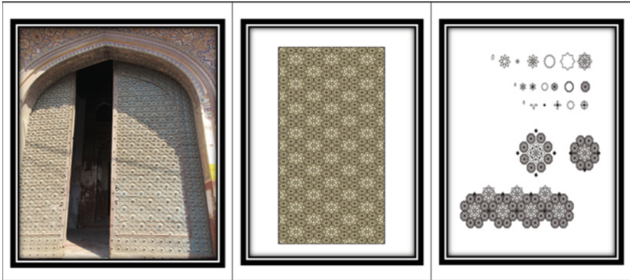
Fig. 18.14 Wooden door of old haveli of Aatma Ram with layout and details (Source: Author)
