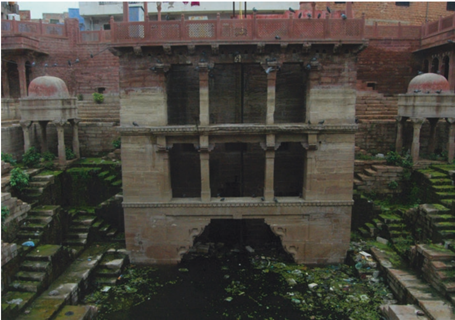
Fig. 8.4 Mahilabaug Jhalara at Jodhpur; like all the other water structures, this beautiful structure lies abandoned and neglected though it continues to provide water to the city. Lack of care has made it a place for garbage leading to a loss of water quality
