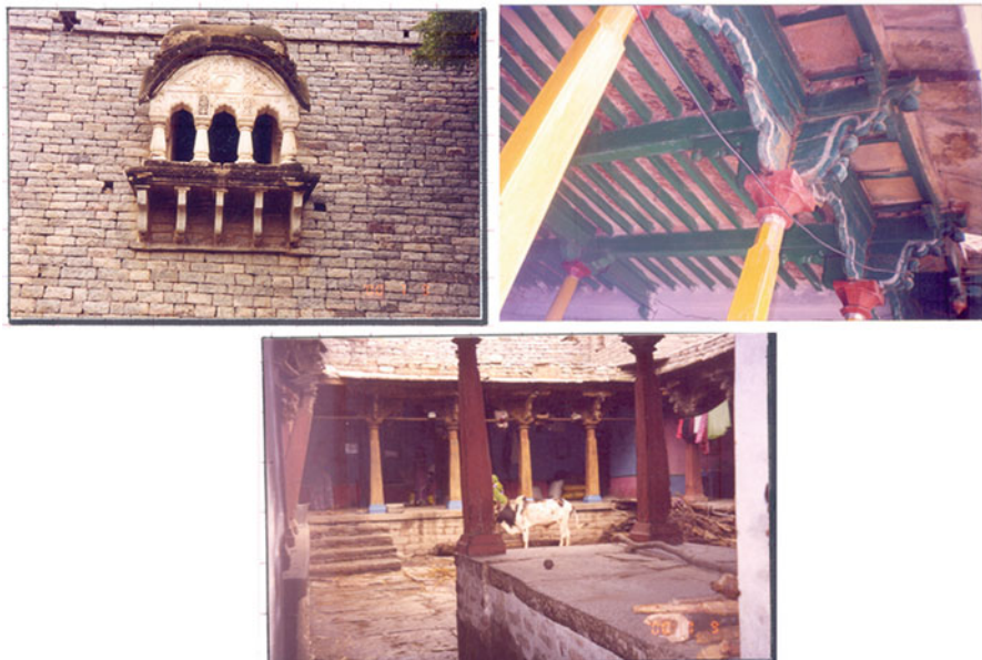
Fig. 12.7 Shows use of materials and construction techniques used in walls, roof, and floor
