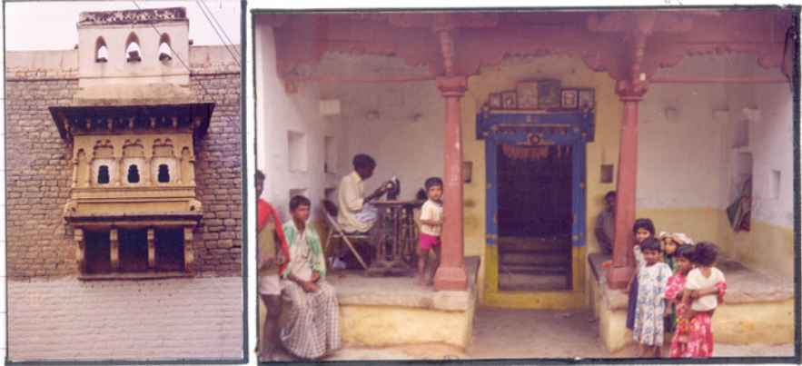
Fig. 12.13 Shading devices are used to protect from heat penetration
