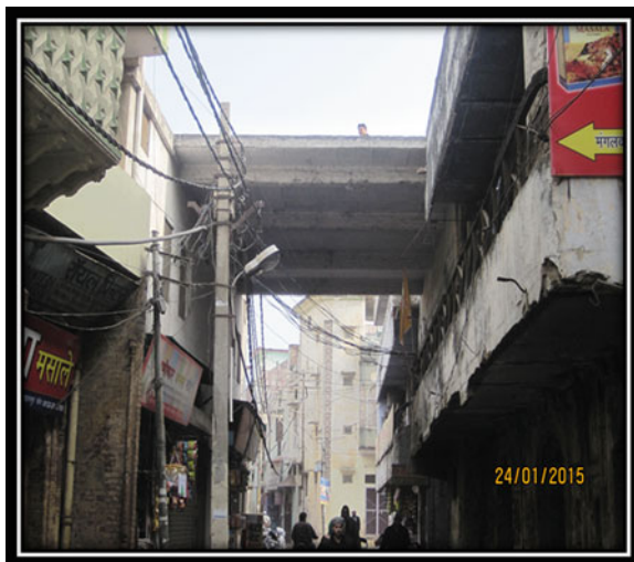
Fig. 18.6 A general view of chhatta Jambudas (Source: Author)
