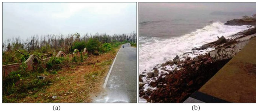
Fig. 10.13 (a) Casuarina shelter belt that survived the onslaught of Hudhud. (b) The broken staircase leading to the badly eroded beach at Kirlampudi Layout, Visakhapatnam
