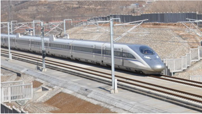
Fig. 10.9 Slab track of high-speed railway at the subgrade section
