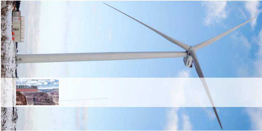
Fig. 1.3 Crazy architecture versus routine in wind turbine design: cantilevering structures. The large photo shows the horizontal axis wind turbine Vestas V164-8.0 MW ® installed at the Østerild wind turbine test field, Denmark, with a tip height of 187 m, a hub height of 118 m and a blade length of 80 m [62] (photo credits: Frank Boutrup Schmidt). The photo is rotated by 90° (and mirrored) to illustrate the structural challenge of withstanding the aerodynamic loading of the turbine rotor. The small inset photo, set at approximately the same scale, shows the Skywalk Grand Canyon cantilevering 21 m from the canyon wall (photo credits: Fabrizio Marchese)
