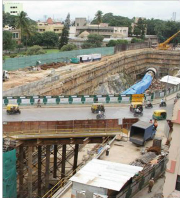
Fig. 12.6 Underground twin tunnel TBM construction near Kalasipalyam, Bangalore. (a) North-south alignment, (b) east-west alignment
