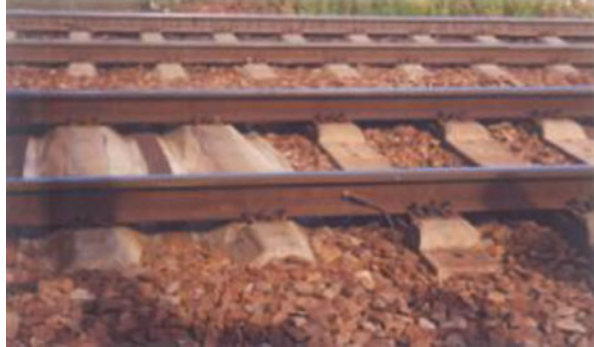
Fig. 7.2 Ballasted track with wide sleepers
