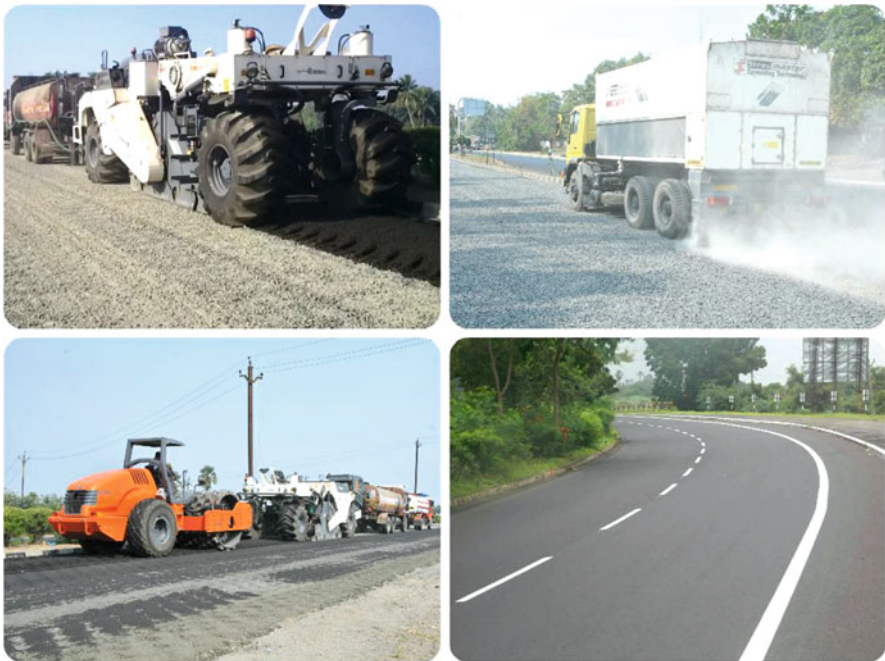
Fig. 3.5 Various stages of cold in-place recycling at Baroda-Halol section (Wirtgen 2012)
