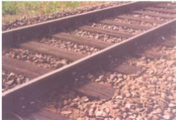
Fig. 7.1 Ballasted track with timber sleepers
