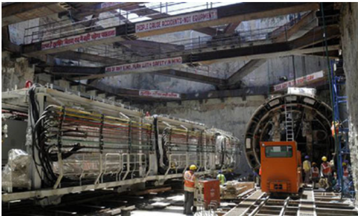
Fig. 12.12 Tunnel boring machine (TBM) (Ref: http://www.thehindu.com/news/cities/chennai/life-of-a-metro-the-first-look-underground/article3502044.ece )
