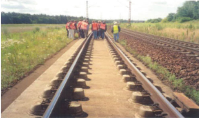
Fig. 7.3 View of a slab track in Germany
