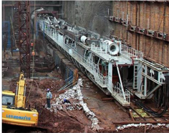
Fig. 12.9 Tunnel boring machine which is assembled for a length of 96 m begins the tunneling work (Ref: http://www.delhimetrorail.com/whatnew_details.aspx?id=c4kjd1nWTgMlld )
