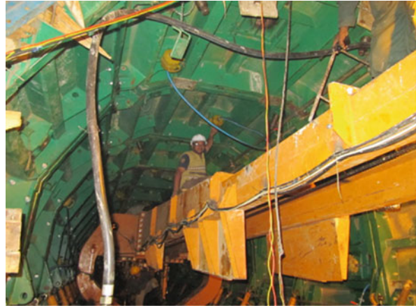
Fig. 20.4 Tunnel lining formwork
