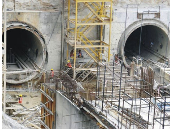
Fig. 12.11 Twin tunneling work at Washermanpet, Chennai Metro (Ref: http://www.masterbuilder.co.in/the-tunneling-heroes-of-indian-metros/ )
