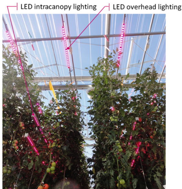
Fig. 16.1 Overhead and intracanopy SL from LEDs for tomato plants grown in a greenhouse
