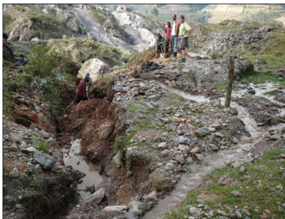
Fig. 10.1 Diverted water stream. Photograph Diverted water stream (Macháček 2012)
