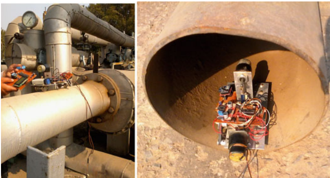
Fig. 3 Crawler runs externally and internally on horizontal pipe
