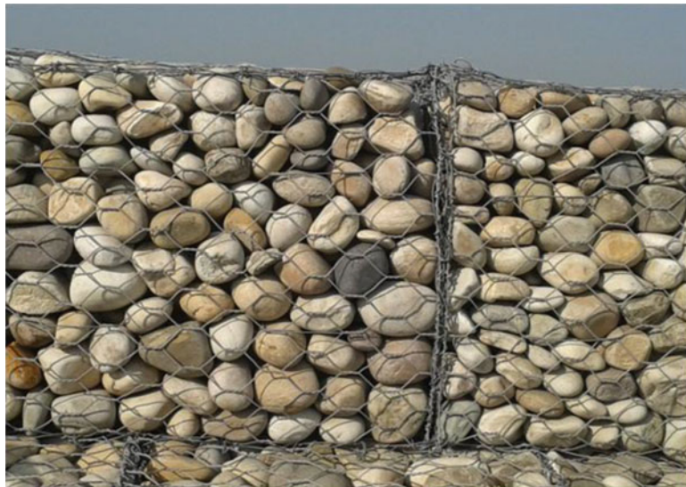
Fig. 15.14 Trail dykes made of gabions using manufactured D.T. hexagonal wire crates
