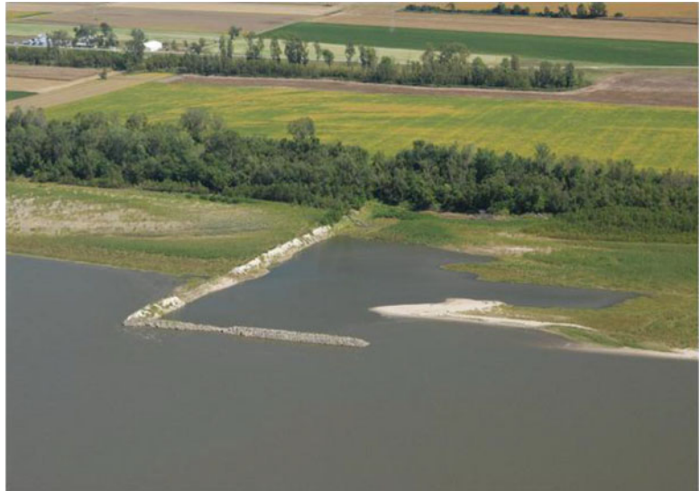
Fig. 15.15 Sedimentation around trail dykes on the Mississippi River
