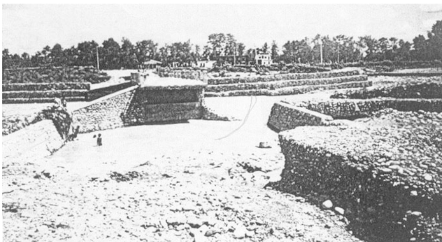
Fig 14.2 Outflanking of a vented causeway on the stream ‘Danab Khola’ in Nepal
