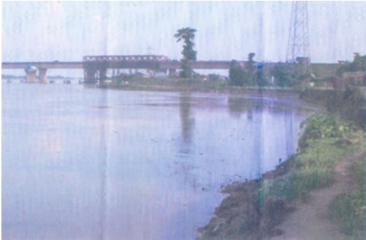
Fig. 14.11 Embayment of right bank of River Mahananda u/s of Mahananda Bridge on NH-31
