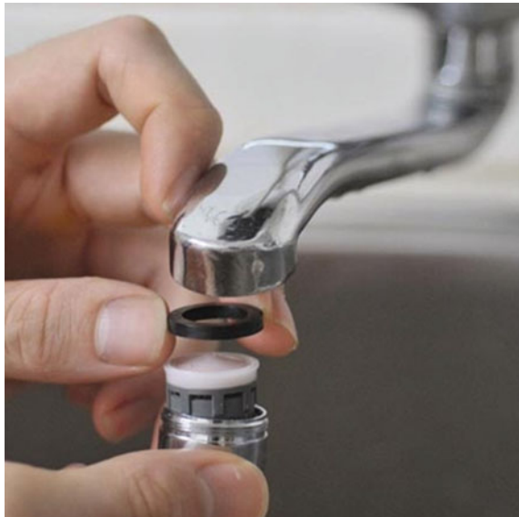
Fig. 8.1 Photo showing an aerator fixture at a water faucet (DrainWorks 2014)
