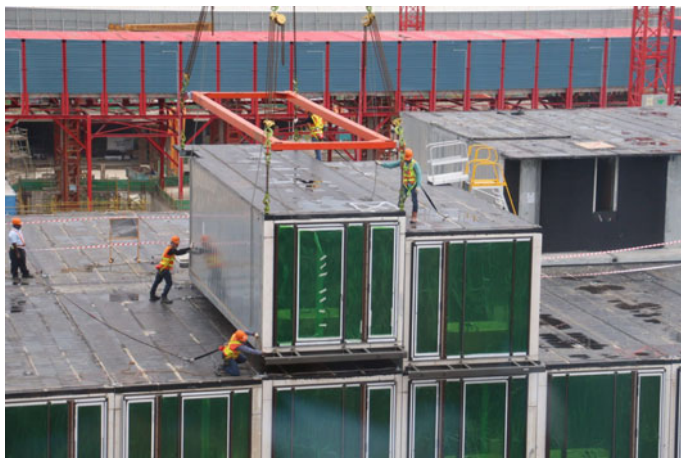
Fig. 8.10 Site photo of a PPVC assembly in Singapore
