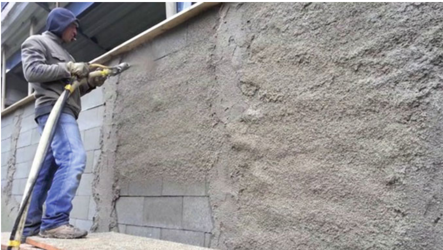
Fig. 4.9 Photo showing application of a thermal insulation plaster (MagorTherm 2015)
