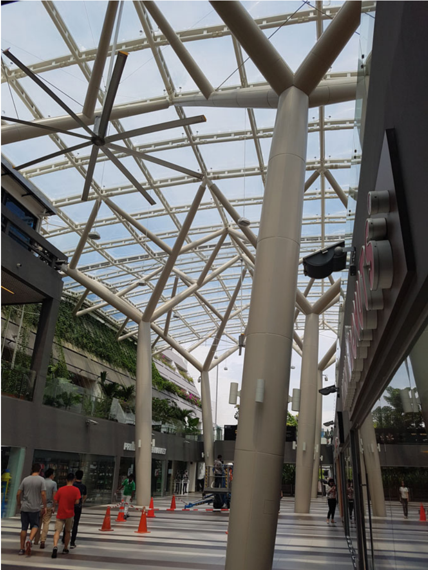
Fig. 4.21 Photo of a skylight installed above an open walkway in a building
