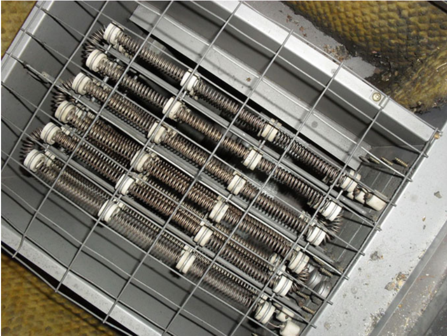
Fig. 5.2 Electrical heater resistor coils used in a electric boiler (Kristoferb 2016)
