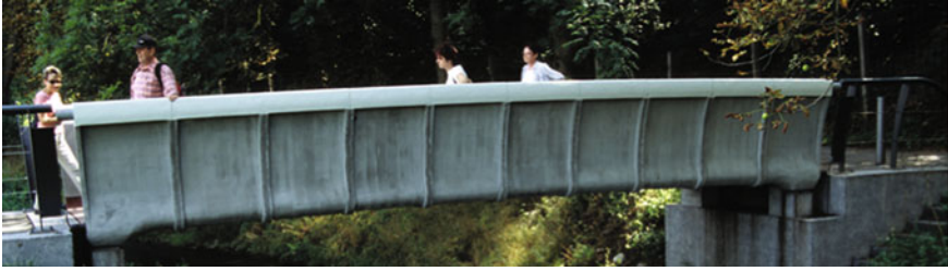
Fig. 1 Pedestrian bridge at Oschatz, Germany, made from TRC, by courtesy of SFB 528
