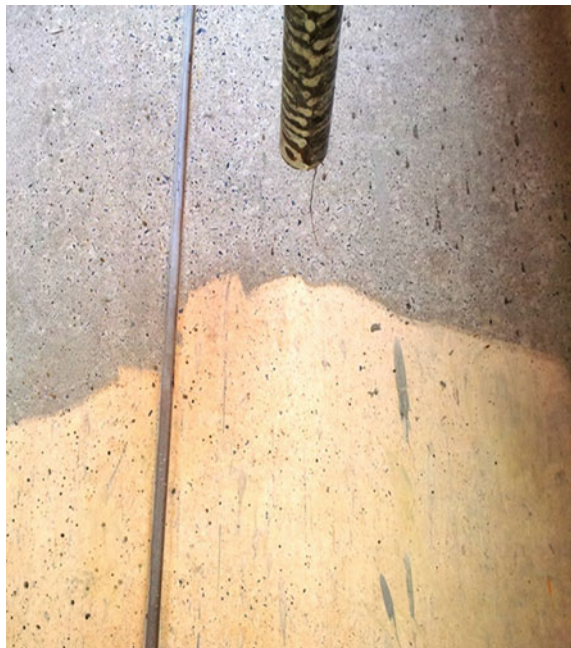
Fig. 8 First step of cleaning: washing with hot water. Source Authors, 2013
