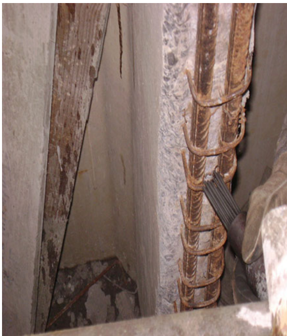
Fig. 10 Reinforcement cleaning using needle gun. Source Authors, 2013
