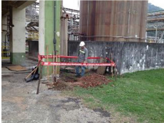
Fig. 19 Excavation spot on an isolated area
