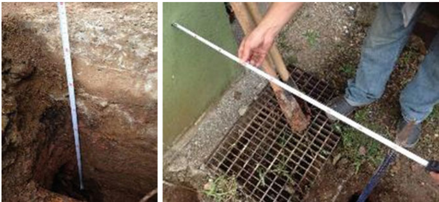
Fig. 21 Measurement of the foundation structures dimensions
