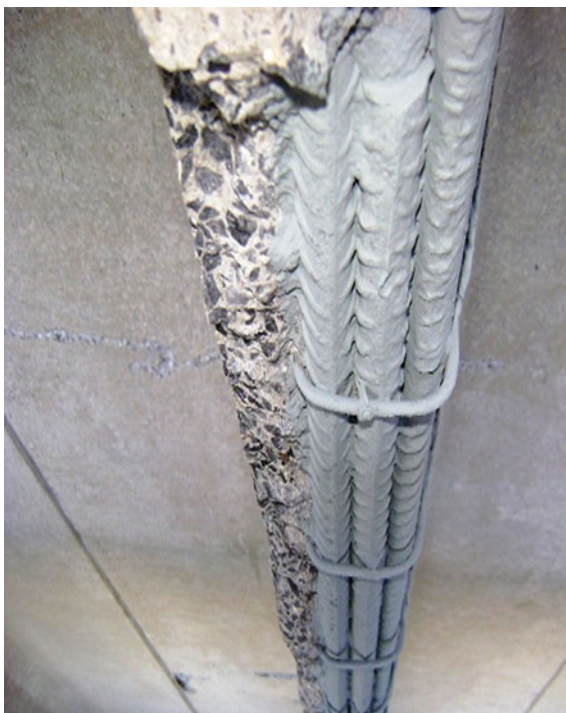
Fig. 12 Application of epoxy rich zinc for reinforcement protection. Source Authors, 2013
