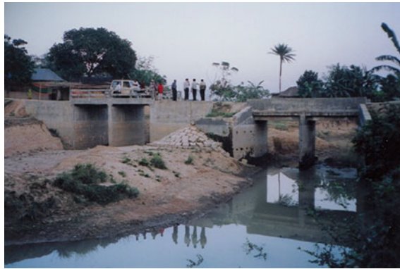
Fig. 4 Drainage improvement of Dhodrar River at 18.0 km
