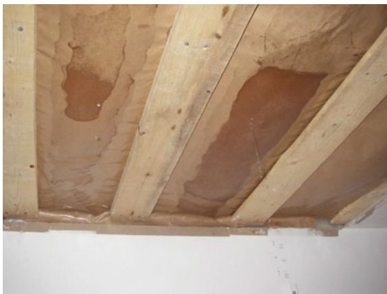
Fig. 4 Example of leak in a roof assembly detected during a moisture performance assessment
