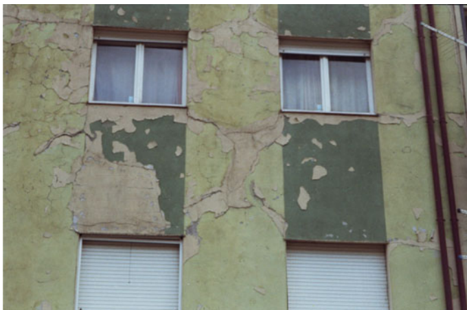
Fig. 2 Wall facing west
