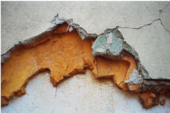
Fig. 1 Building with ETICS in PIR in Torrette di Mercogliano (Avellino). Insulation thickness: 3 cm; cementitious render: 2.0–2.5 cm; finishing coat: paint
