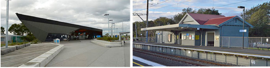
Fig. 15.3 Images of two railway stations on the South Morang line
