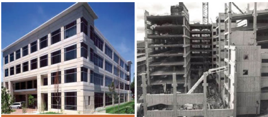
Fig. 1 IBS precast wall in building constructions
