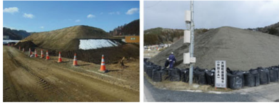
Fig. 1 Tsunami deposit soils placed in the stockyards
