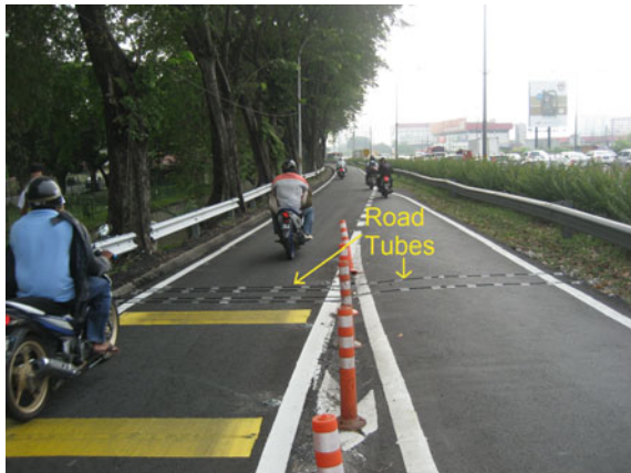
Fig. 4 Place where tubes of ATC are located at Site 1
