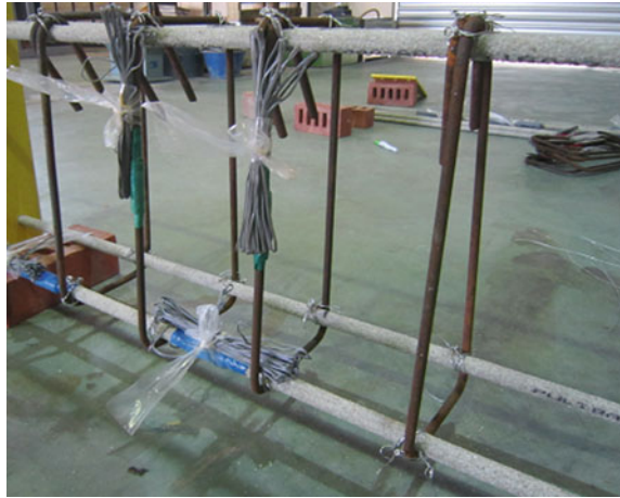
Fig. 1 GFRP bars as longitudinal reinforcement
