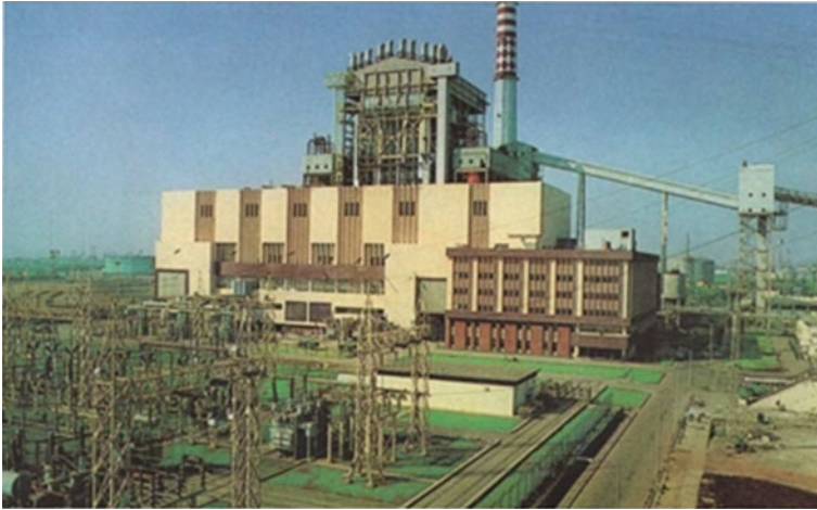
Fig. 3 500 MW thermal power unit at Trombay
