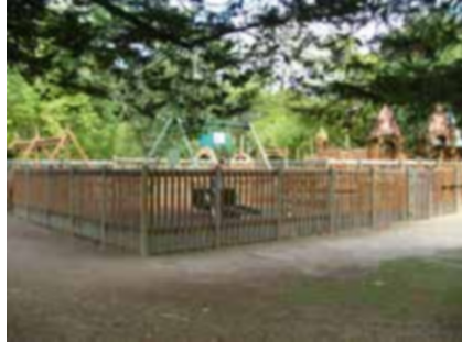
Photograph 4. The Liberty Swing is located on the periphery facing away from the playground
