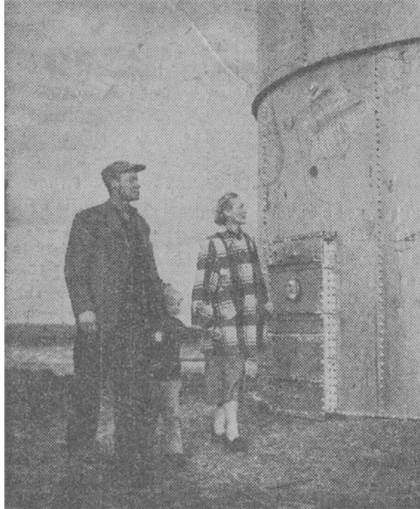
Figure 9.3. Elsie, Bill, and Claudia inspect a crude oil storage tank (© 1953, Winnipeg Free Press).
