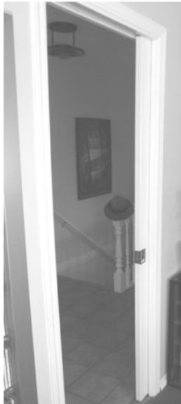
Fig. 11.9 A pocket door is only about 35 mm thick and slides in a pocket of 45 mm width.
