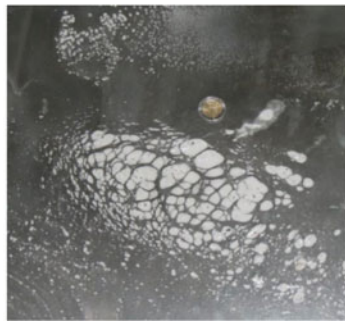
Fig. 3.5 Case-study glass footbridge: (a) live loads; (b) steel tendon and (c) local delamination
