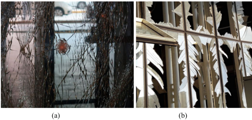
Fig. 3.2 Examples of damaged glass facades after the tragic attacks at (a) Istanbul and (b) Brussels airports
