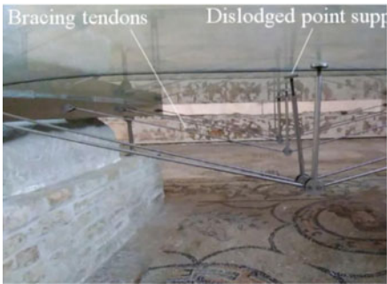
Fig. 3.5 Case-study glass footbridge: (a) live loads; (b) steel tendon and (c) local delamination
