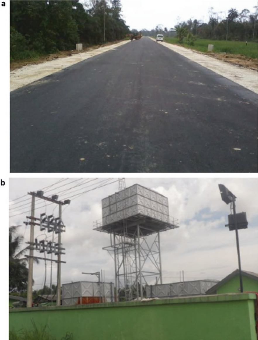
Fig. 14.6 (a) 4 km road built between Shell's facilities and Gbaran host communities (Gbaran/Ekpetiama cluster). (b) Water tower for the Gbarantor community (Gbaran/Ekpetiama cluster). (c) Power station for Obunagha and Gbarantor communities (Gbaran/Ekpetiama cluster). (d) 18-classroom block in Onopa community (Epie/Atissa cluster) (Source: Shell)
