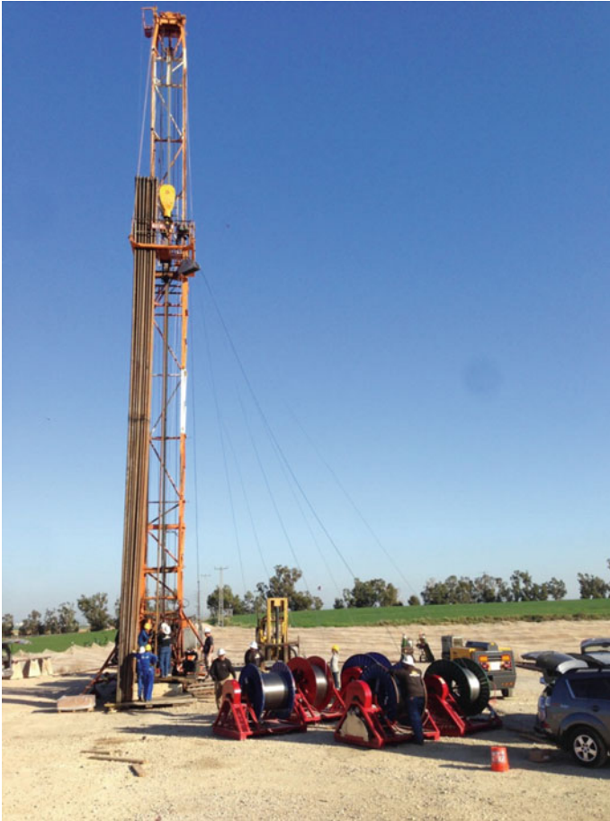
Fig. 8.9 Workover operation in progress at H18a showing rig with double stands of tubing and pneumatic spooling units used to tension control lines as they are fastened to the tubing
