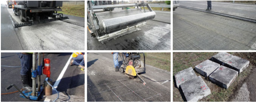
Fig. 1 Application of a pre-bituminised grid and sampling procedures for laboratory tests
