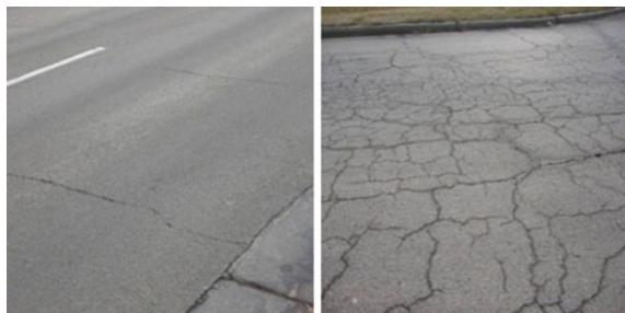
Fig. 1 Thermal cracking ( left ) and block cracking ( right ) on asphalt concrete pavements in Illinois
