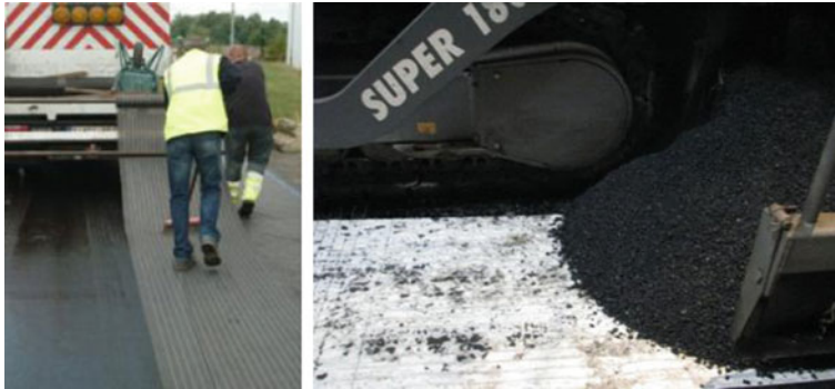
Fig. 1 Installation process of the new flexible steel-based anti-cracking interlayer
