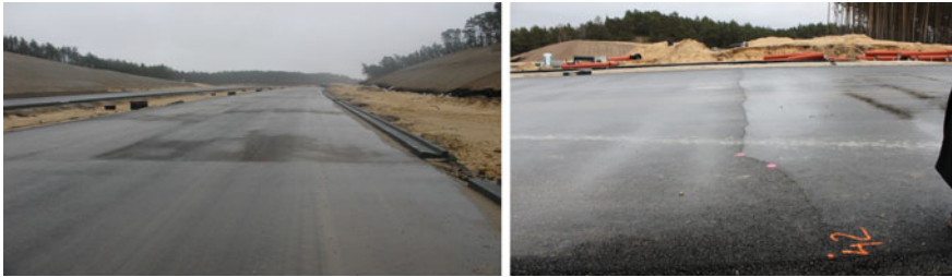
Fig. 1 Examples of the HMAC base with non-homogeneous surface texture
