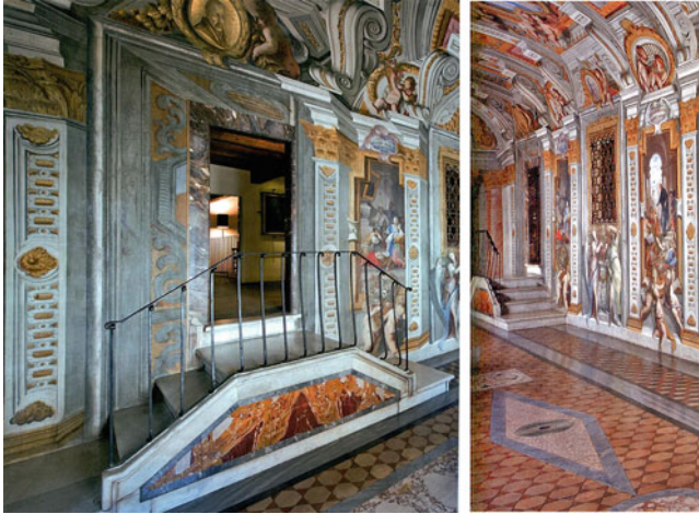
Fig. 21.8 Pozzo's new communication door. ( left ) View from the Corridor. ( right ) Grated window references as "L" in Fig. 21.7 [2]
