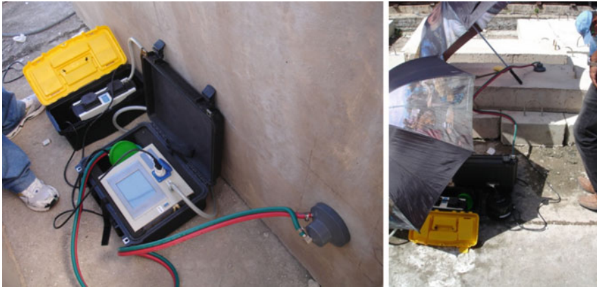
Fig. 2 Measuring kT on one culvert (l.) and on one Block C1 (r.)
