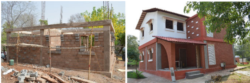
Fig. 4 Various stages in construction of demo building
