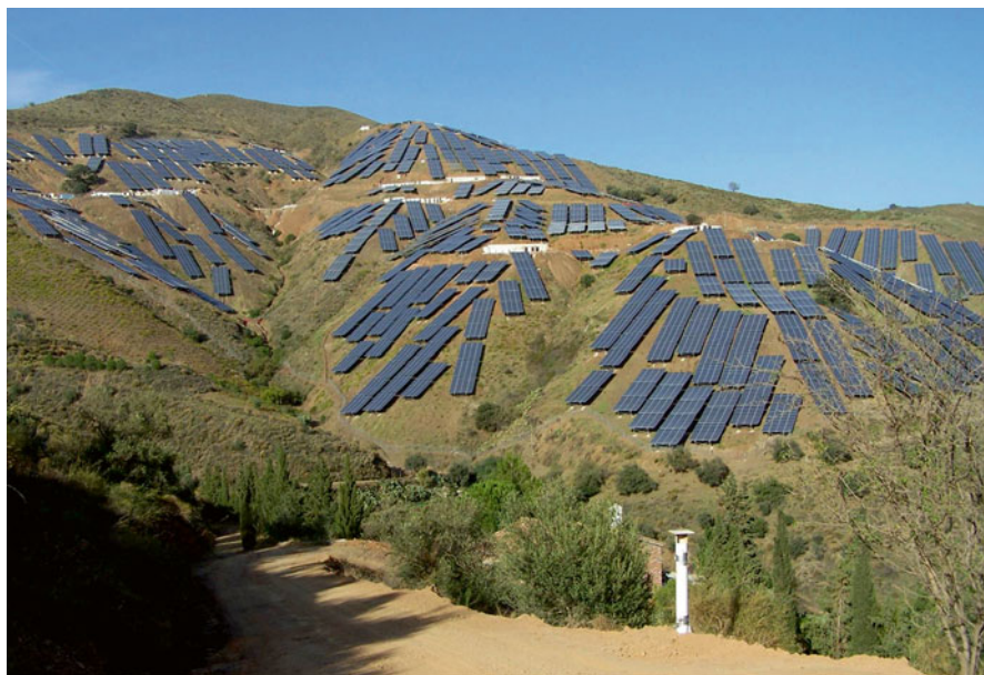
Fig. 14.3 Landscape impact of photovoltaic power plant in mountain area (Moclinejo, Málaga province)
