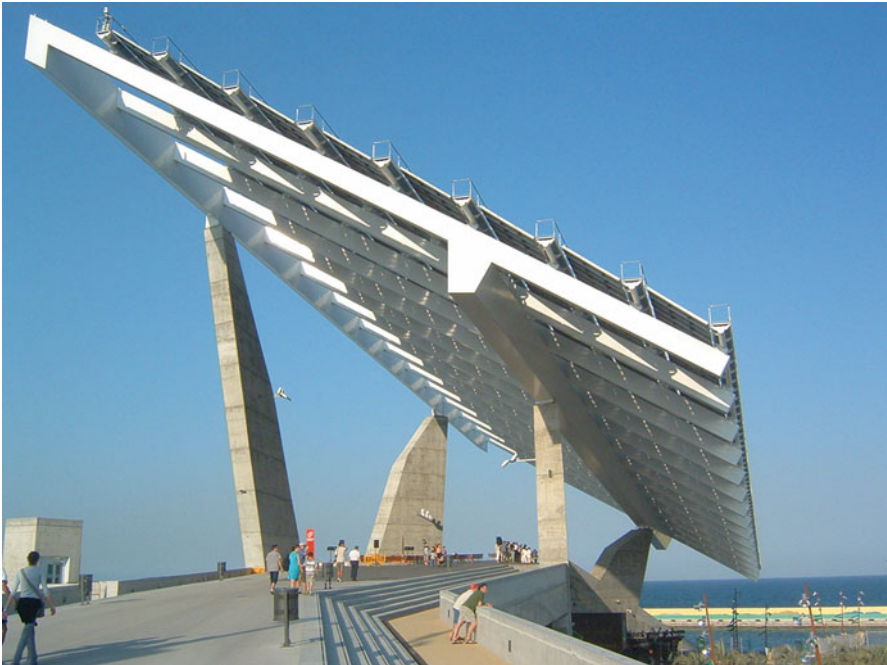
Fig. 4.4 PV pergola in the venue of Barcelona Forum 2004 (Source: The authors)
