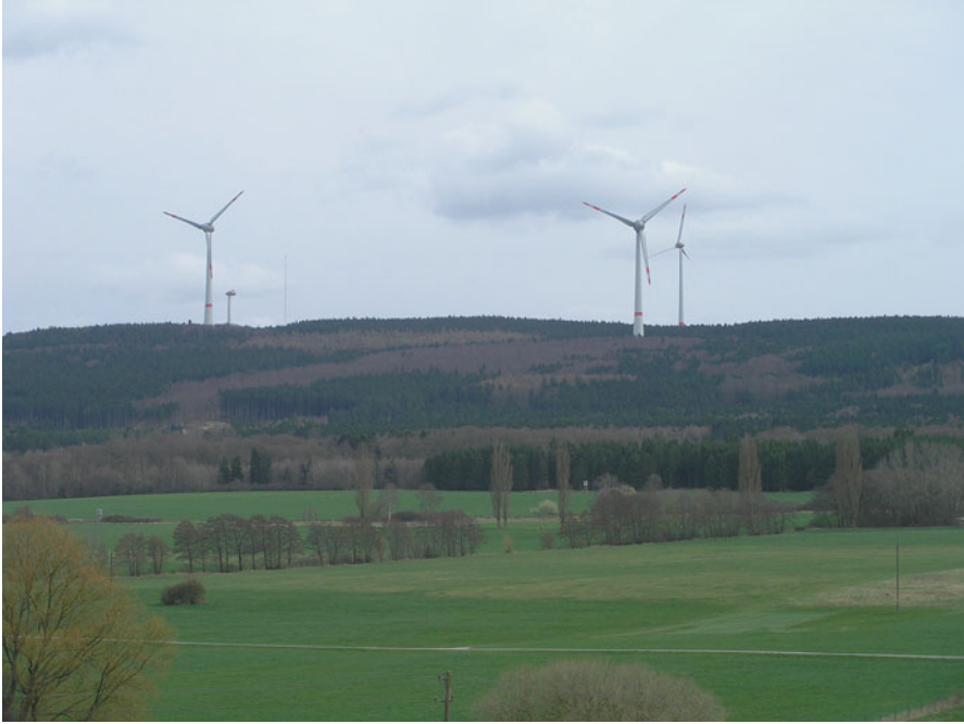
Fig. 12.2 Ellern wind farm, installed in the Soonwald Naturpark (Rhineland-Palatinate) in April 2013
