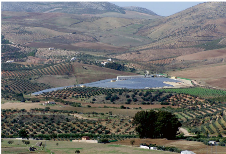
Fig. 14.4 Photovoltaic power plant adapted to plots of land (Ardales, Málaga province)
