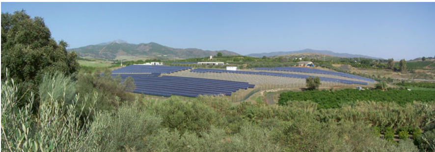
Fig. 4.3 Solar farm located in the Province of Malaga (Andalusia) (Source: The authors)
