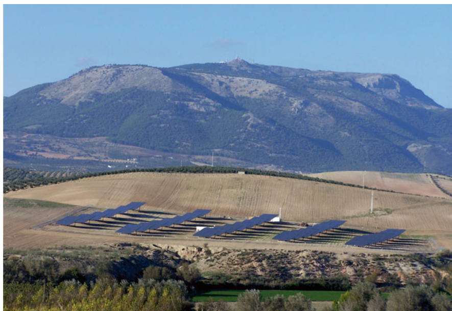
Fig. 14.2 Trackers in photovoltaic power plant (Fuensanta, Granada province)
