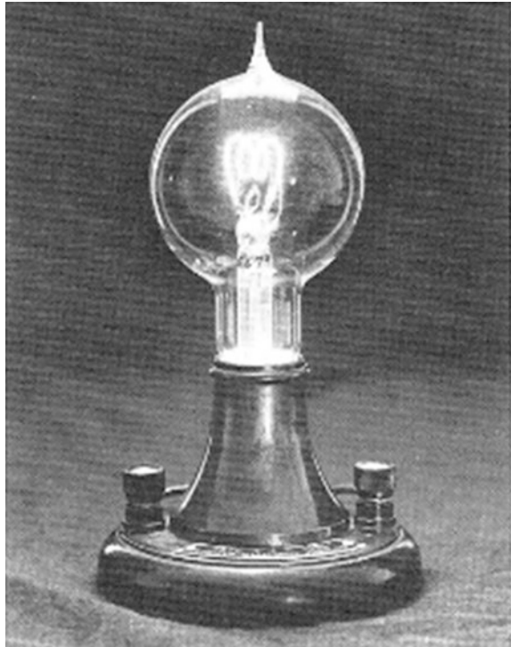
Fig. 1.7 Replica of Edison's first electric lamp containing a carbon fiber filament [15]
