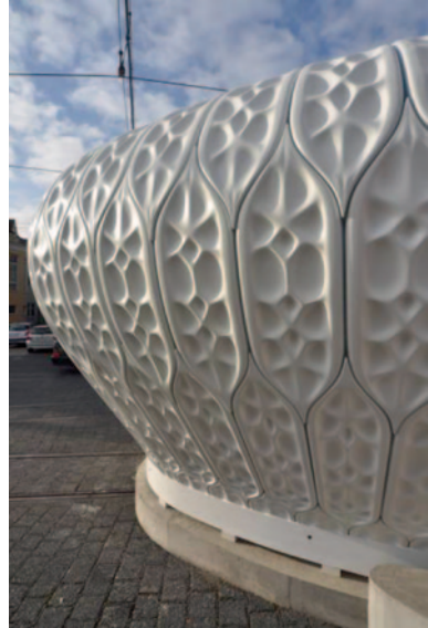
Fig. 5.11 The research structure COCOON_FS showing a modular structure composed of a restricted number of building block types reminiscent of the highly repeated patterns in diatom valves. Note that the assembly process of COCOON_FS differs radically from the way diatom frustules are formed. http://www.pohlarchitekten.de ; http://www.planktontech.de (© G. Pohl)
