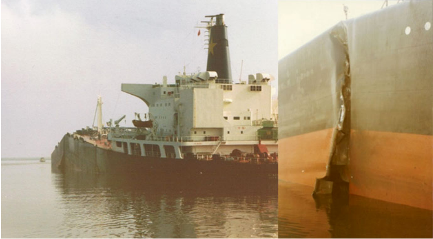
Fig. 12 Vessel structure that failed because of overstress in hogging (Source: Cornelius de Keyzer, Master Mariner, Port of Rotterdam, the Netherlands)
