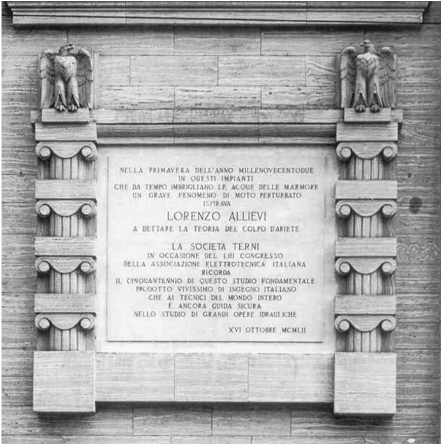
Fig. 5 The marble plaque acknowledging Allievi's contributions to the water hammer at Papigno plant in Terni
