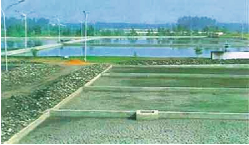
Fig. 15.2 Sewage treatment plant (oxidation/waste stabilization ponds) at Saharanpur, Uttar Pradesh, India
